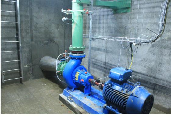
Fig. 5. Centrifugal PaT installed in the technical room next to the lower reservoir.
