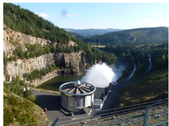
Fig. 7. View of Naussac II power-house.
